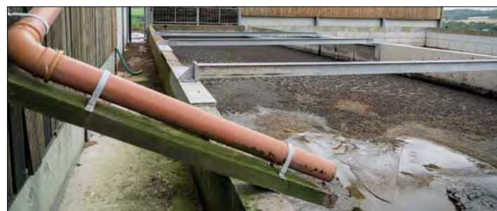
Slurry is separated to allow for easier handling and nutrient utilisation
