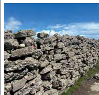
Ex-airfield runway concrete walls
