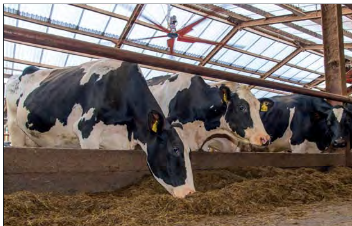
Plane Tree Farm installed heat reflective roof panels and ceiling fans
